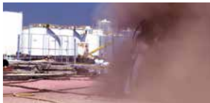
Conventional abrasives can create excessive dust
